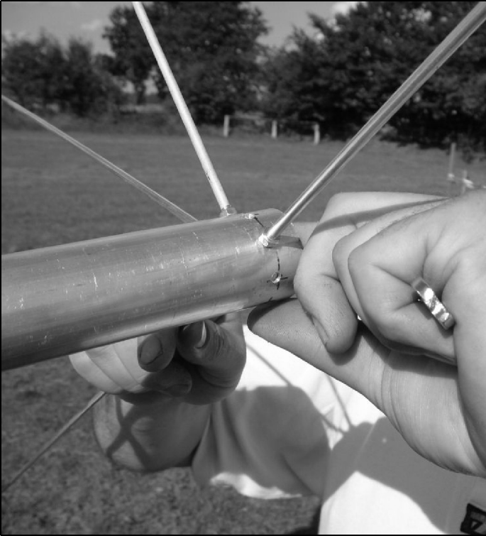
Fig. 8: The assembly of the individual aluminium rods at the end of the tube for the top load.
