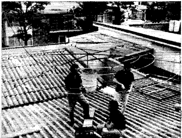
The "circular cylindrical" antenna shown above (1.) was constructed by Raul Mejia M., HK4TA. He reports that the antenna performs well, is resistant to high winds and bad weather. The circular elements are made from 1/2-inch aluminum tubing and are formed on the ground. The lengths are determined by using conventional formulas for quad element lengths. The photograph on the right shows HK4TA, HK4PJ, and HK4BAJ adjusting the antenna with a grid-dip meter and a communications receiver.
