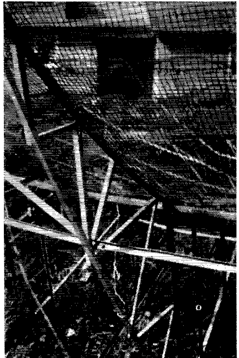
W3SDZ used hardware cloth for the covering on his 432-Mc. dish. Note the construction of the struts and supports.
