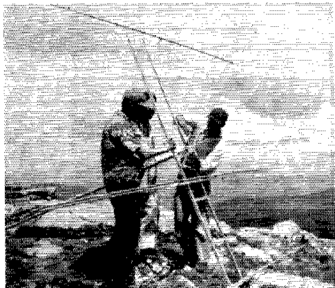
Atop picturesque Mt. Spokane (elevation 5800 feet), three of a crew of 17 Spokane Radio Amateurs wrestle with a ten-meter beam installation for W7NBR/7.
