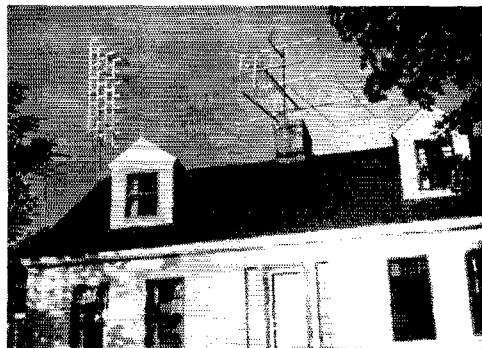
Antenna systems at W1RFU, Wilbraham, Mass., northern end of the 410-mile 420-Mc. record contact with W4TLM of Yorktown, Va. The 420-Mc. array at the left has 64 elements. Horizontal and vertical twin-leads for 144 Mc. and a 4-element array for 50 Mc. are mounted above the chimney.
