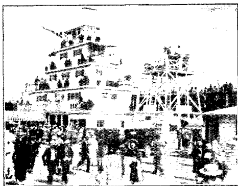
THE ADMINISTRATION BUILDING AND THE KEY STATION AT THE BASE OF THE MOTION PICTURE PHOTOGRAPHERS TOWER
