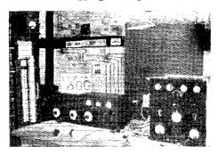
CANADIAN 3GG. The Edison Storage batteries that supply the plate circuit, with the charge-discharge switch and plate voltmeter, are seen at the left of the picture.
