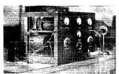
Portable Transmitter NKF-1. Wave length range 66 to 115 meters. This set frequently works IXAM, South Manchester, Conn. (about 300 miles) In daylight with antenna 20 feet high. 9XAX has been worked easily on reduced power.
