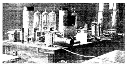
The transmitter at NKF. 250-watt master oscillator feeding three 250-watt power amplifier tubes. Plate input 1500 watts from 1000-volt storage battery. This set puts an earsplitting 50-meter signal into 1XAM by daylight during all weather conditions. On 50 meters the signal is better than on any wave between that and 110 meters.
