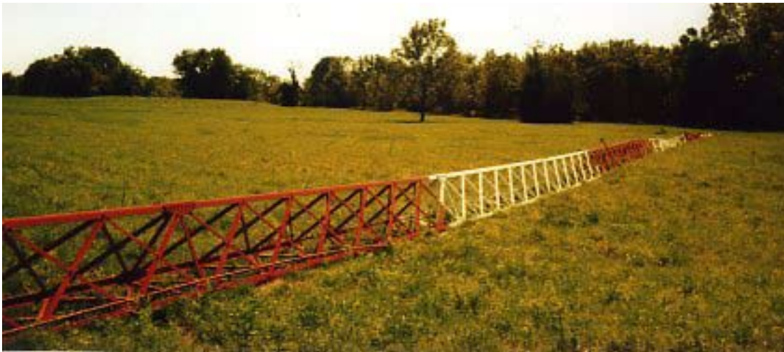
A WAEB-790 tower lies prone after vandals cut a guy wire to it.
