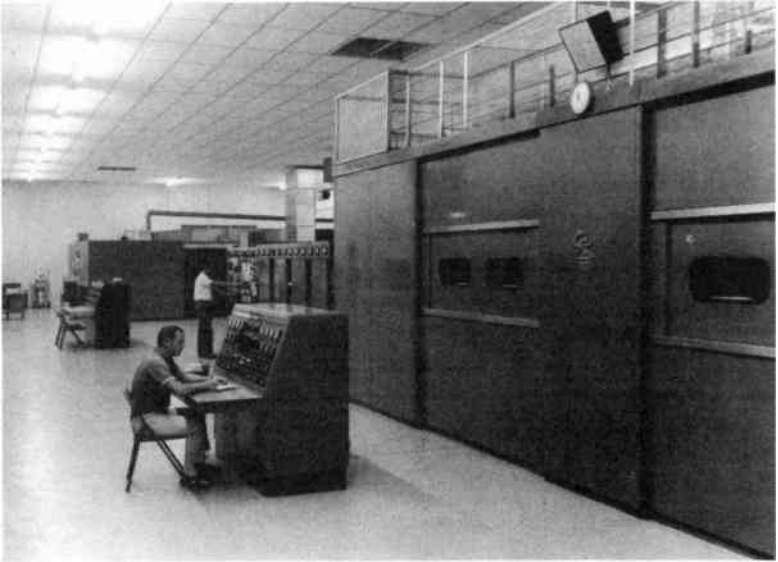
Fig. 1-5 This is Transmitter Hall at Trans-World Radio in the sunny Netherlands Antilles. TWR's huge 500kW (800kHz) AM broadcast transmitter is shown being monitored from the foreground console. A 260kW shortwave broadcast transmitter is being adjusted in the background. (TWR photo)
