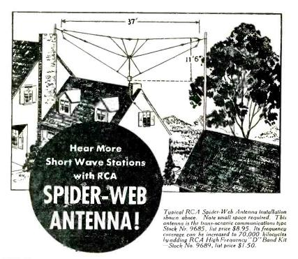
ERE'S an antenna that makes it easy for you to tune those "hard-to-get" stations! The RCA Spider-Web Antenna System gives excellent signal pickup over a frequency range from 140 to 25,000 kilocycles. If you wish, this coverage can easily be stepped up to 70,000 kilocycles.
