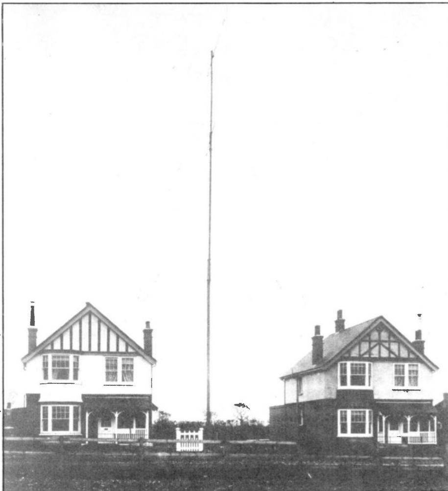
How things were 'way back then' in 1901, the 120ft mast towers above the two houses which were home to the wireless school.
