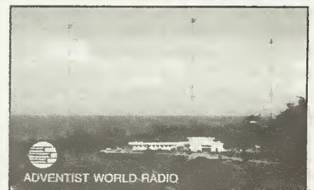
AWR Asia's transmitter building and first antenna system on Guam. There are now three more towers.
