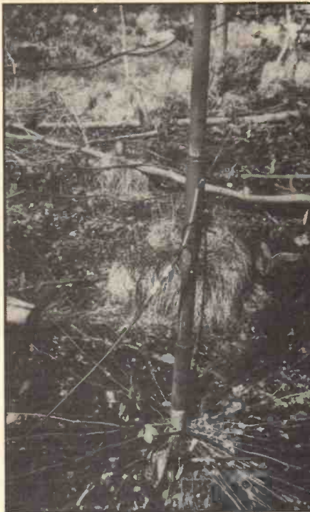
The radial system at the base of a vertical used in a 4 ele vertical array at W1CF illustrates good engineering practice for such a system. In addition, the array is located in a swamp further enhancing ground conductivity.
