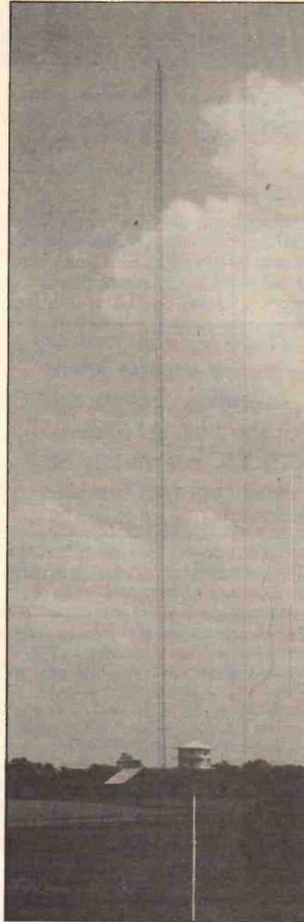
A \frac{1}{4} wave vertical for 160m at N4AR. Currently there are two of them in phase.
