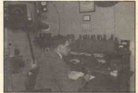
Austrian EACM in his shack in 1927. Top left is his 400W single valve self-excited transmitter. The receiver on the desk was an early superhet.
