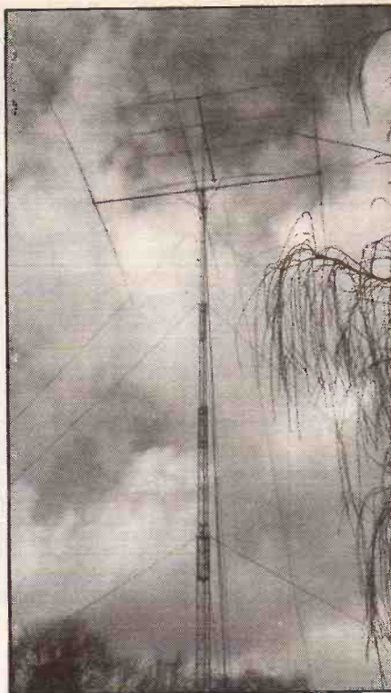
The antenna system at GB2PX a KT34 4 ele triband beam and a KLM 3 ele 40m beam up 90'.
