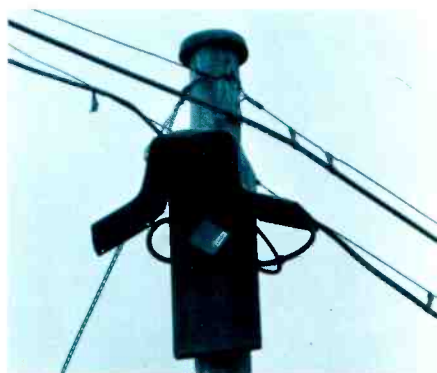
Directional coupler used in Chichibu system has 300 ohm output to subscriber. Drops are twin lead or ladder line.
