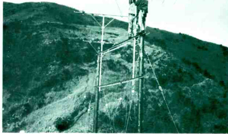
Technicians are shown completing the head-end installation for the Hakone system.
