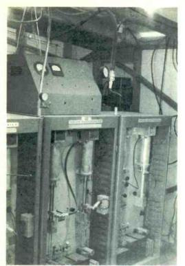
INSIDE THE TRANSLATOR SHACK three Adler units crank out the UHF signals from the two Los Angeles stations and a Tijuana, Mexico station.
