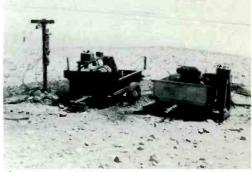
SO REMOTE is the Palm Springs translator site that all power must be "trucked in." The original generators were run on butane, while this pair operates from gasoline hauled to the top of the desolate peak.
