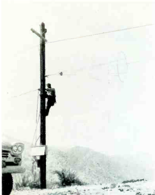
Installation of Ameco perfected G-line system in Antennavision's Glove-Miami system.
