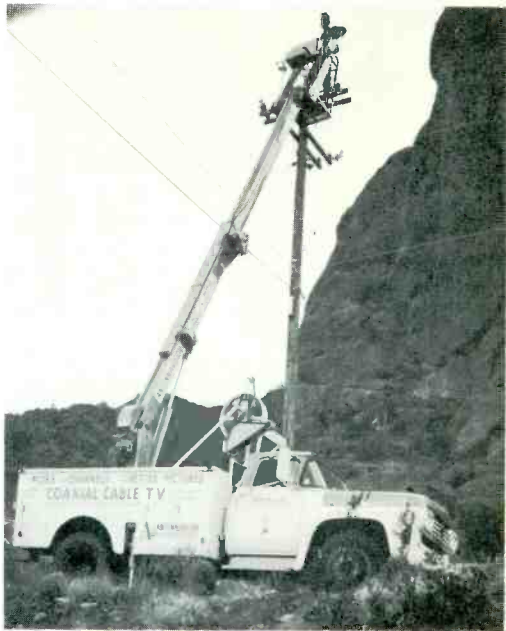
Antennavision's $18,000 aerial line construction truck shown in operation during construction of its Paradise Valley system in Phoenix, Arizona.
