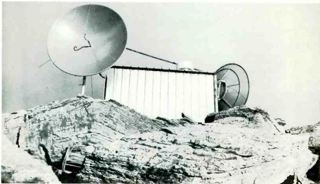
Microwave relay point on Preston Mesa which receives four Phoenix TV channels from microwave transmitter on Hutch Mountain and transmits to microwave relay point at Jacks Peak for delivery to Antennavision's system at Glen Canyon Dam site at Page, Arizona . . . 250 air miles from Phoenix.
