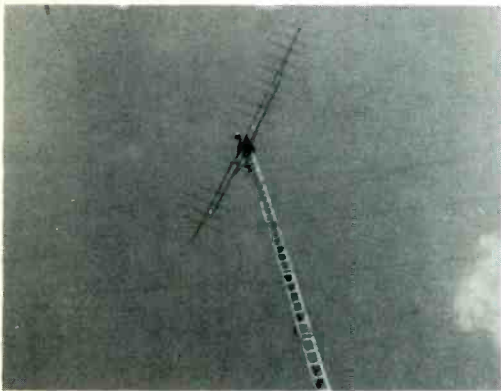
ERNEST V. BLAIR and his 30 foot long-john yagi, 100 feet in the air. Ernest is the small dot on top of the antenna. Parachute anyone?
