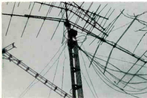
STEEL TOWER all over and through the roof line in Modesto! In the foreground, the smashed mid-section of the 120 footer. In the background the upright but smashed 80 footer with "totaled" low-high and FM yagis.
