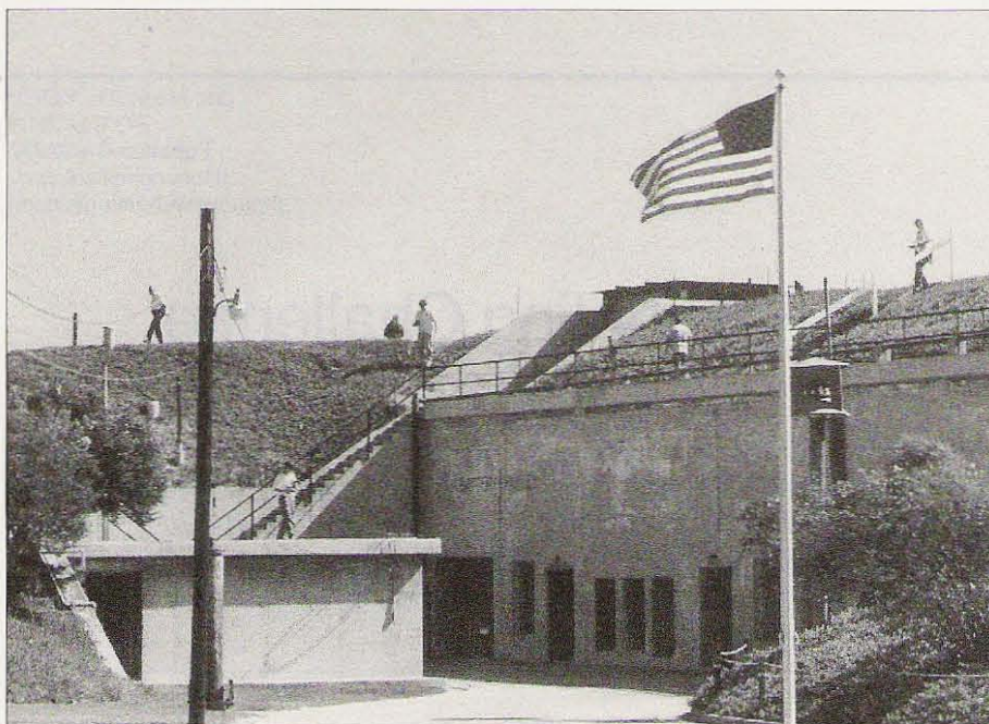
Photo B. Foxhunters swarm over fortifications at old Fort MacArthur during the 1999 Hamcon foxhunt in southern California. There are two concealed microtransmitters in this view. (Photo by Joe Moell KØOV)
