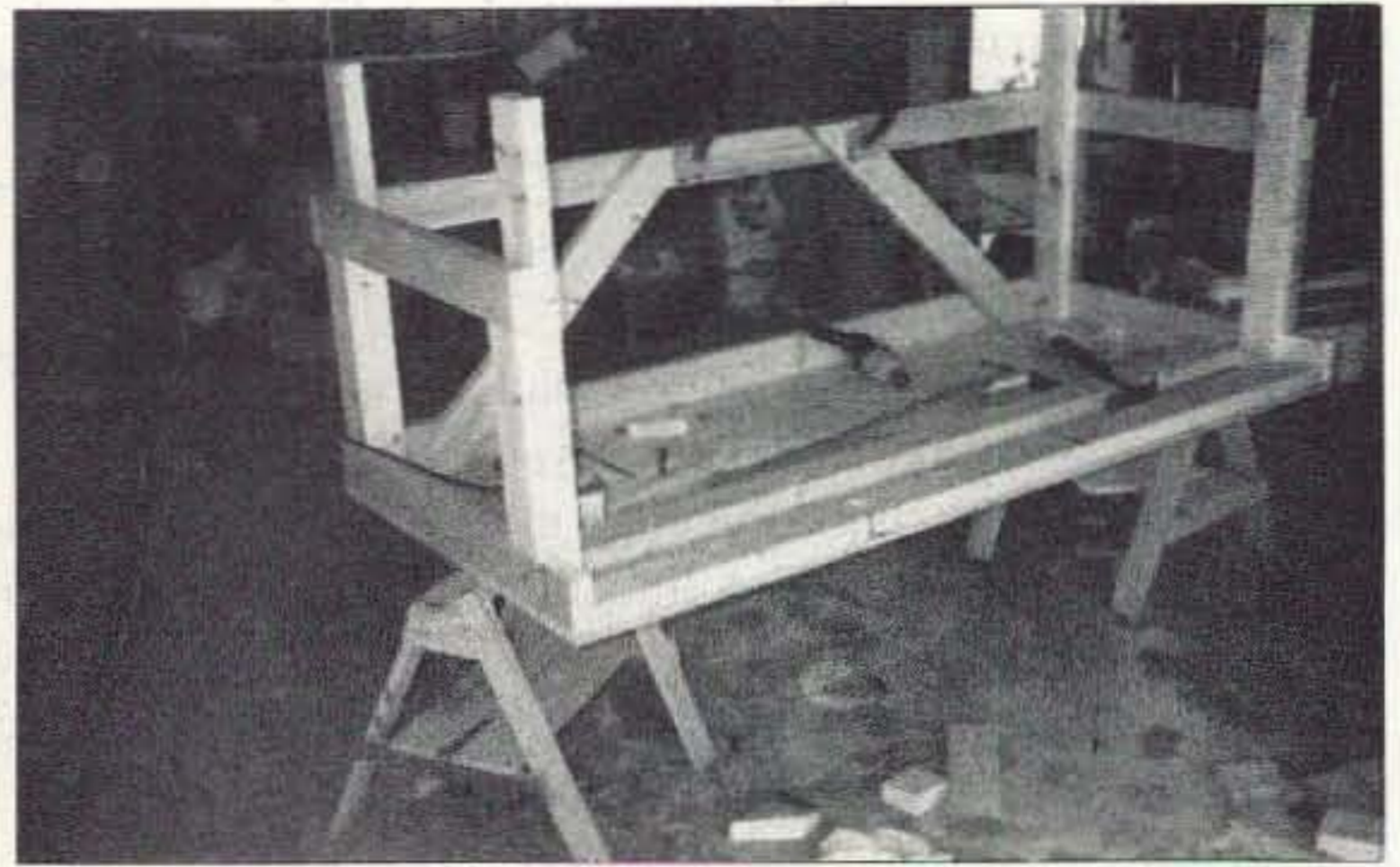
Photo H. Cut the end of a 2-by-4 off to form a 45 degree angle. Place in position as a support, as shown, and mark and cut.
