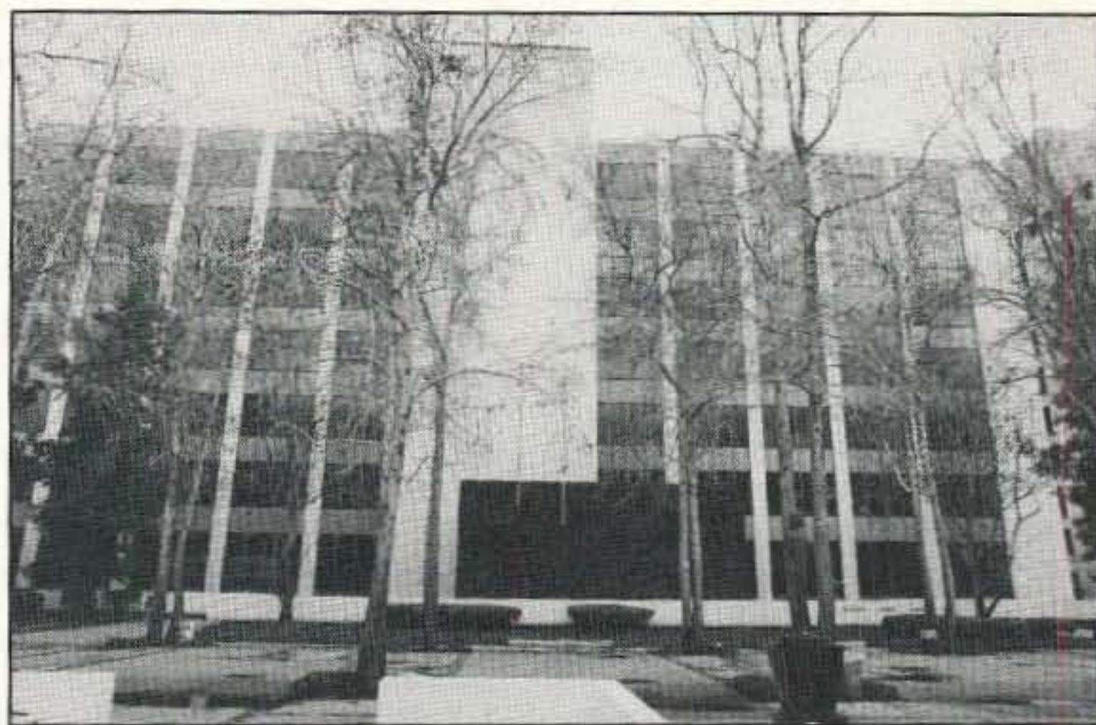
Photo C. The Northwest District Superior Court building is famous for being the site of the recent Menendez murder trial. Now it has another distinction—the source of a signal that jammed sheriff's communications after the Northridge earthquake.
