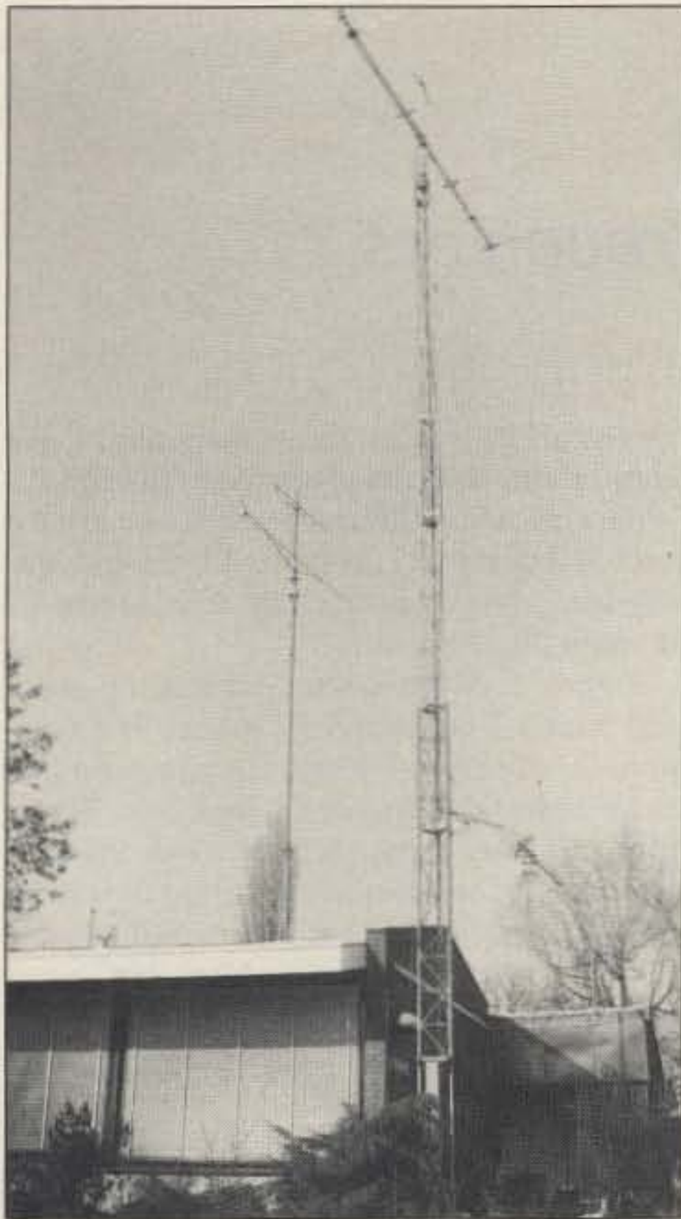
Photo B. JEZ antennas: twenty meter mast with beams for 2 meters and 70 cm; satellite antennas and a Windom above for 40/80 meters; Versatower with DJ2UT beam in foreground. Not visible: Meteosat and ATV receiving and transmitting antennas.
