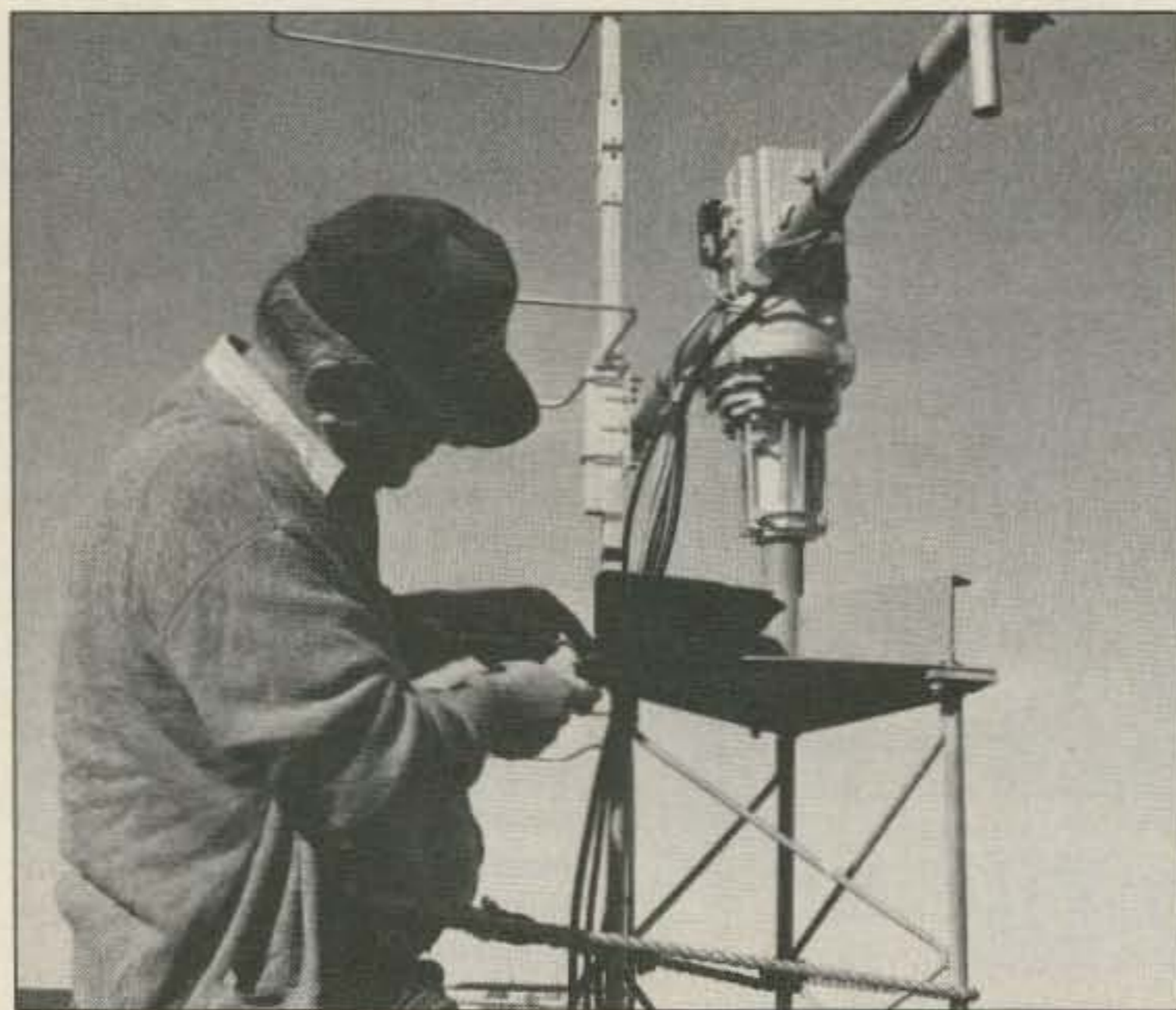
Photo B. KA5ODO secures the tower top plate for the array.
