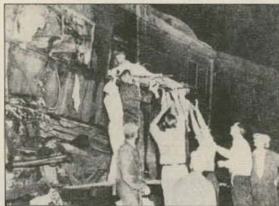
Photo B. The Michigan City wreck required that welders use cutting torches to remove the steel panels from the sides of this Pullman car to free survivors.
