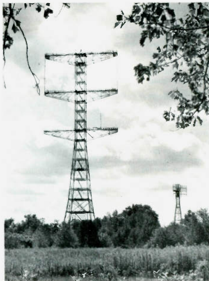
Close-up of the tower. (Photo by Bradley B. Hammond)
