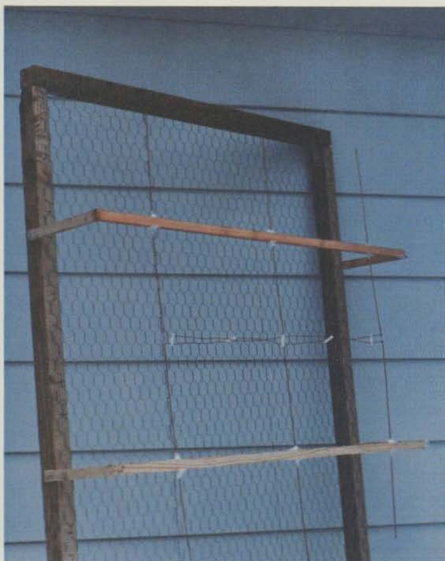
Photo A. Construction details.
