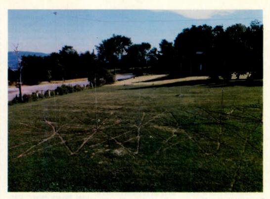
Four more radials were added after this picture was taken, making a total of sixteen; all were from 16 to 20 feet in length. The author employed a trained mole; however, any sharp-pointed garden-weeding or cultivating tool may be used to scratch the shallow trench needed to bury the radial about 1 inch. Refer to Fig. 8.
