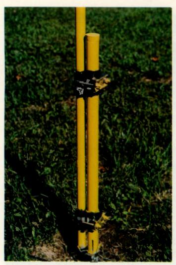
Each of the eight elements is attached to its ground post as shown, using split sections of plastic water pipe for insulators held in place with mylar<sup>TM</sup> electrical tape and clamped together with TV U-clamps. Refer to Fig. 6.
