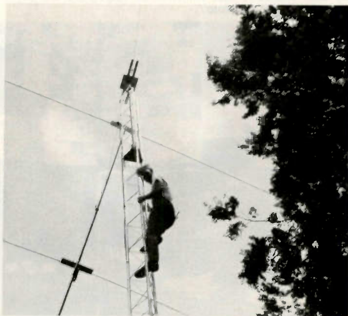
George Lindley WA5HKW erecting his home-brew three-element beam. George built it from plans in Bill Orr's Beam Antenna Handbook for about one-third the cost of a commercial beam. He says it works great.
