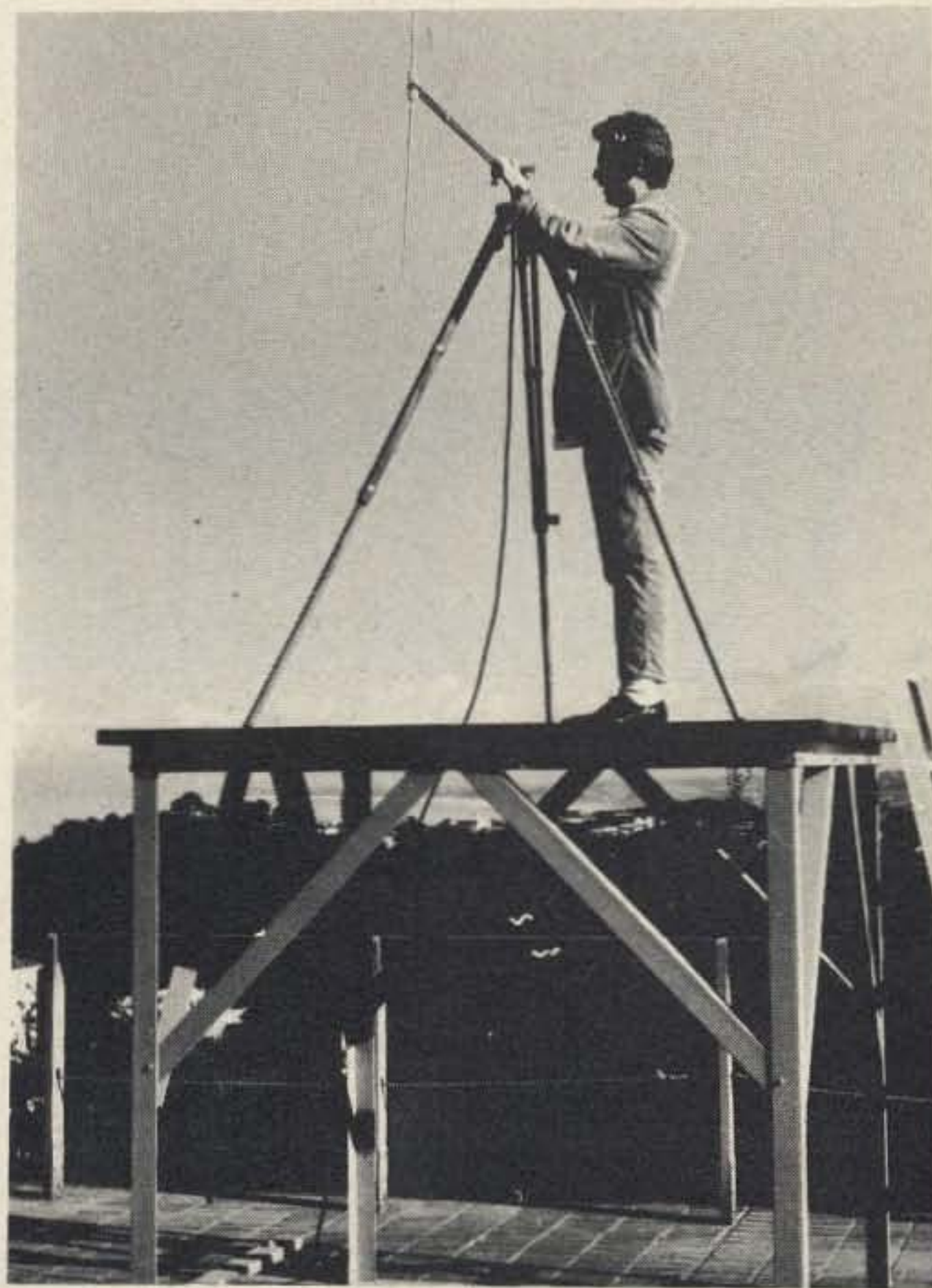
Reference dipole on transmitting platform.
