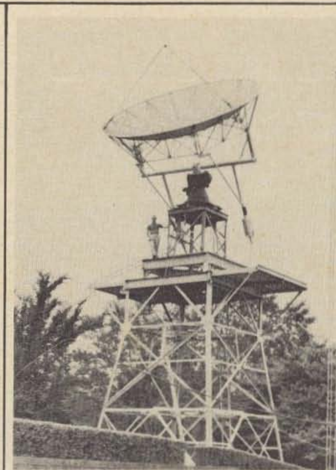
Paul M. Wilson of Collierville, Tenn. stands beside the antenna used in his radio moon bounce experiment. Wilson is a member of the Third US Army Military Affiliate Radio System which provided most of the parts he modified in order to build his imposing radio station.
