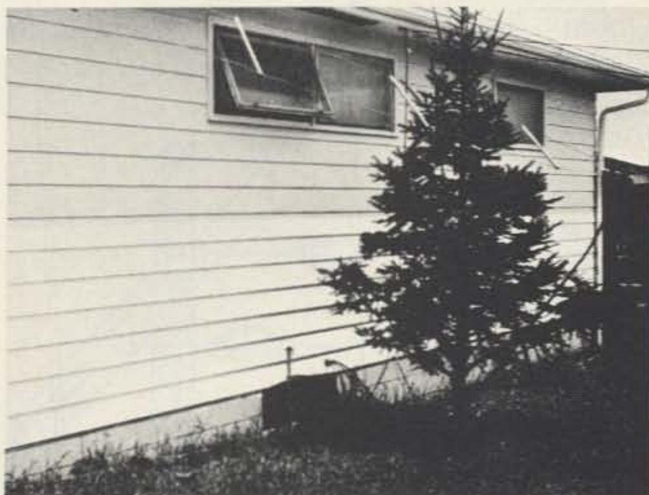
This is the author's method for bringing the ladder line into the shack.
