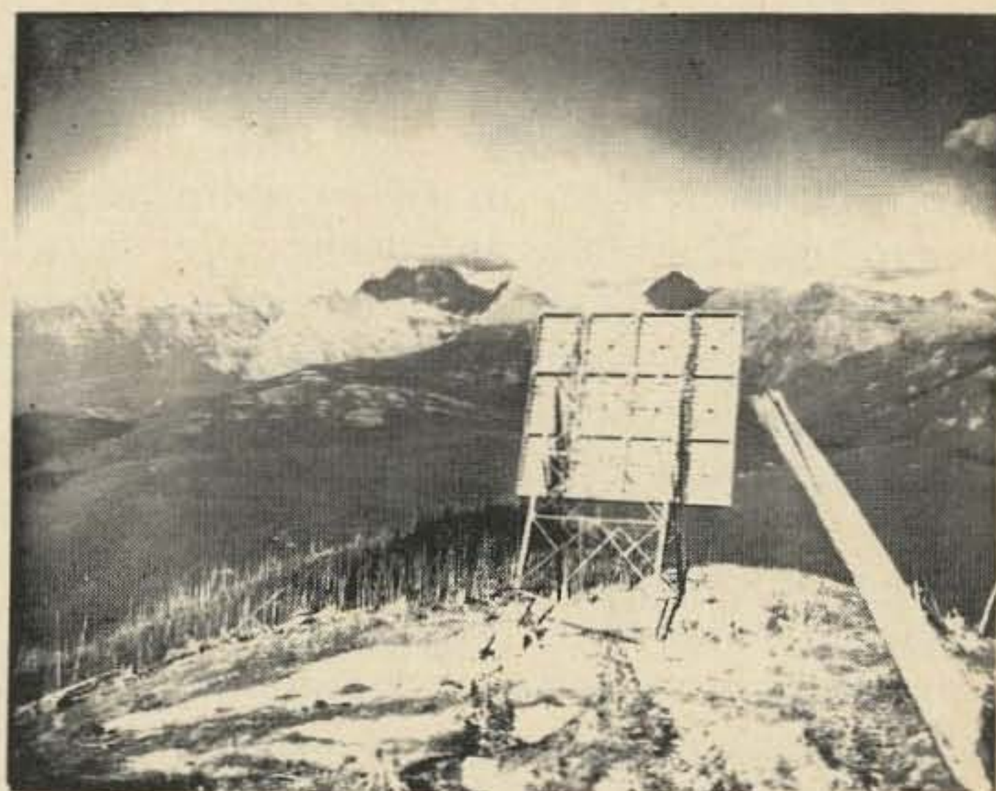
Commercial microwave systems, carrying as many as 960 simultaneous voice conversations or one video program or thousands of channels, use giant radio mirrors such as the one above. (Photo courtesy Microflex Co., Inc., Salem, Oregon.)
