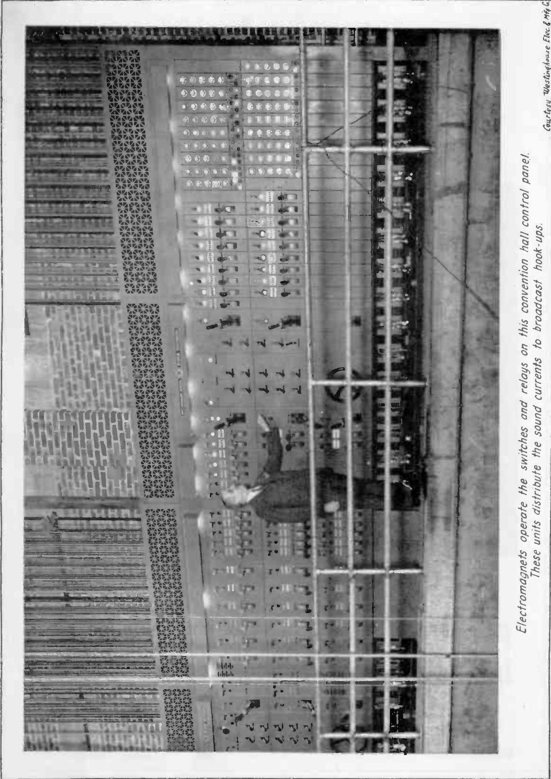
*Electromagnets operate the switches and relays on this convention hall control panel.
