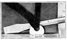
FIG. 45. Method of holding the lace with a screw-driver while tying the final knot at battery tab kk.
