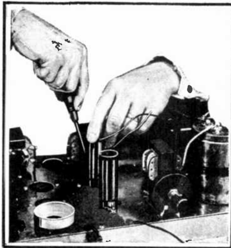
FIG. 1 MOUNTING THE R.F. TRANSFORMER
