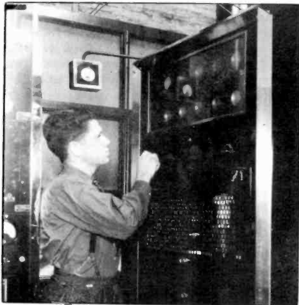
FIG. 1 MODERN BROADCAST A. C. POWER PANEL
