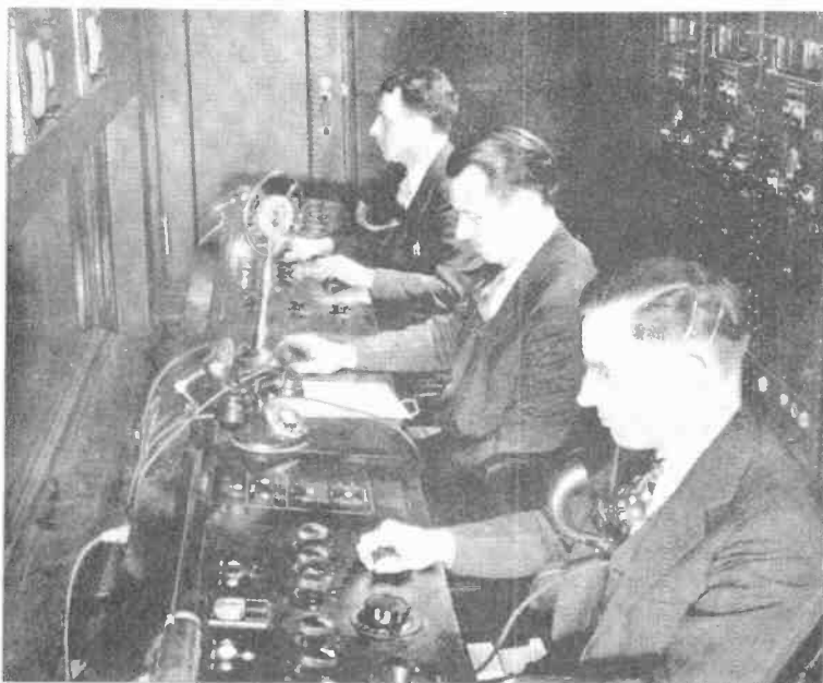
Fig.41 NBC control room.
