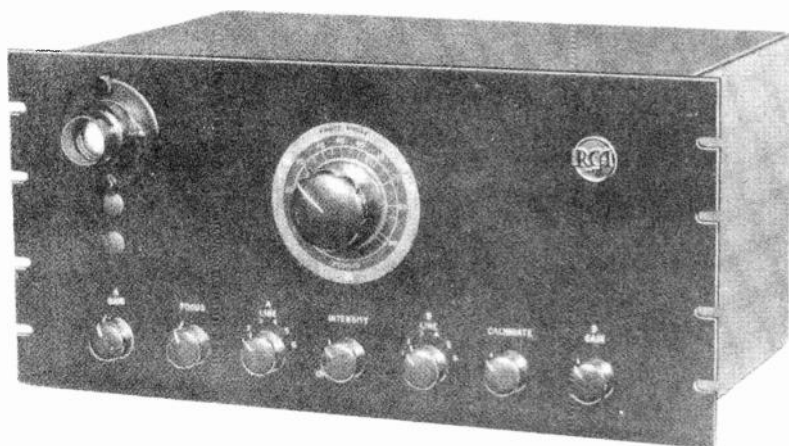
Fig. 15 Photograph of RCA 300-A phase meter.
