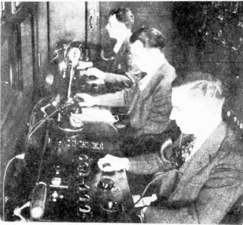
A Modern Television Control Room.
