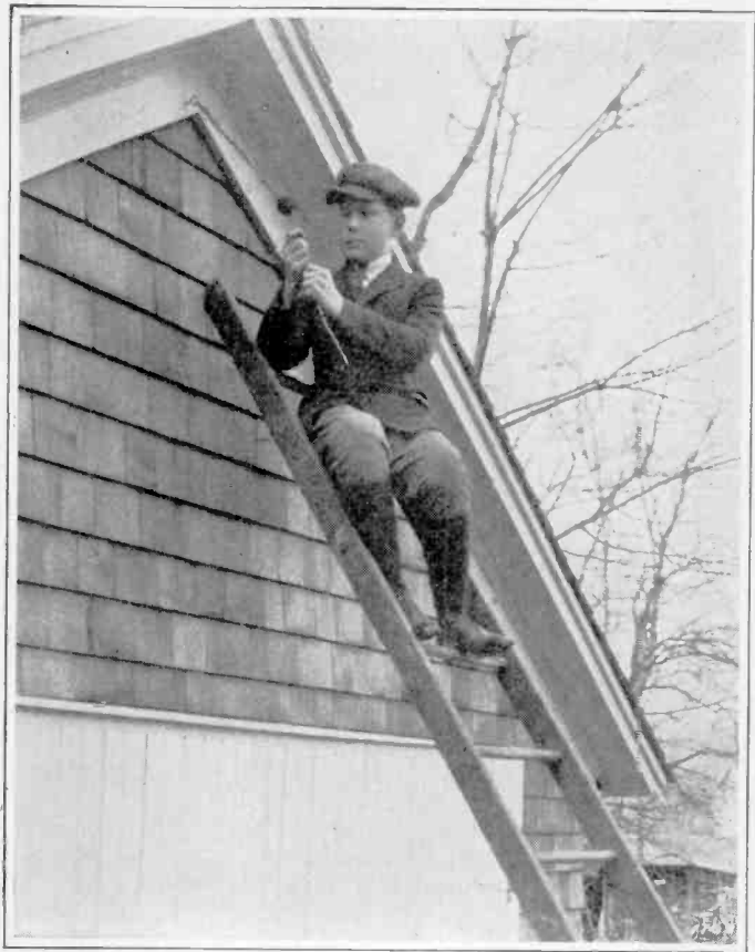
Rigging the antenna.
