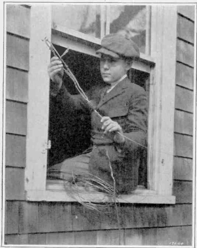
Leading the antenna wire into the house.
