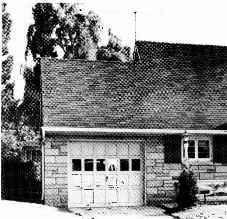
Folded dipole f-m antenna installed on roof of home.
