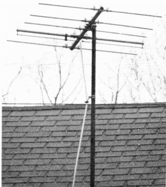
Fig. 1. This is a Yagi type of antenna designed for peak reception on channel 7.
