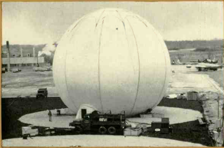
An Air Force tactical radar station, which includes a Paraballoon air-supported antenna, is housed in this air-inflated radome. The enclosed "three-dimensional" radar station on test furnishes range, azimuth, and altitude information for all targets within its 360-degree coverage range. This is a truly mobile, high-power, tactical radar set. All components, including the Paraballoon antenna, can be dismantled into 200-pound pieces.
