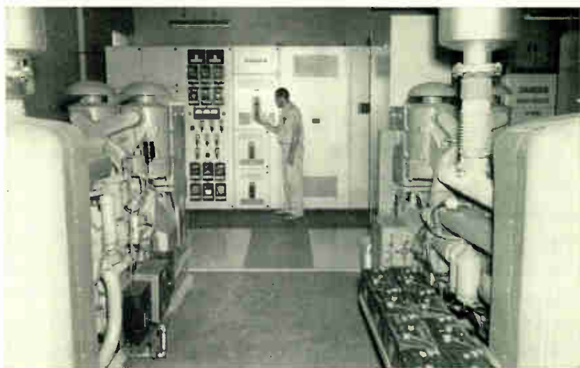
This emergency power supply is designed to meet a critical need. It is located in the County of Los Angeles new Contagious Diseases Hospital unit, which provides services for the treatment of poliomyelitis. For those patients wholly dependent on artificial breathing mechanisms in respirators, doctors estimated that ten seconds was the maximum time that a respirator could be shut down. Thus this power supply is designed for emergency use in the event of power failure. Two diesel-generator sets operate automatically in parallel; power center at the rear is the "nerve center" of the control and distribution system.
