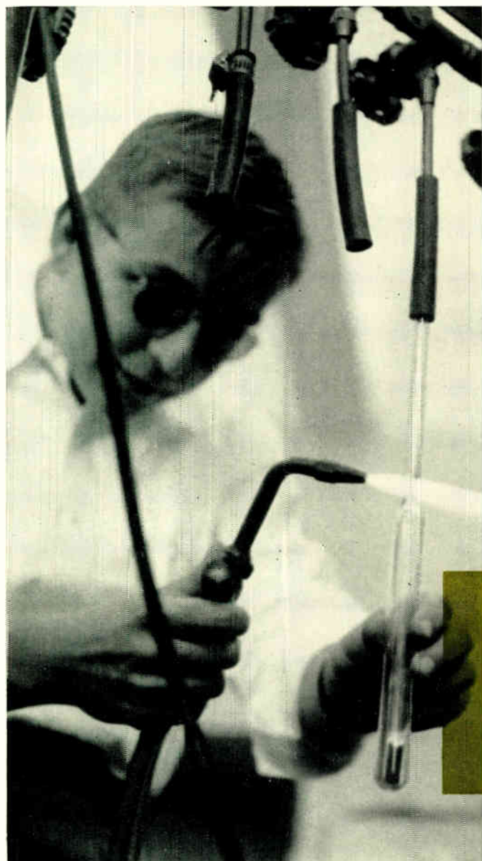
Material to be "baked" is sealed inside a container under vacuum.
