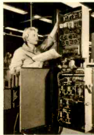
Fig. 11—The automatic bus-duct welder; Cypak cabinet is at top, relay control cabinet is below.
