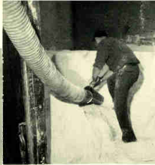
Silos for Clay
