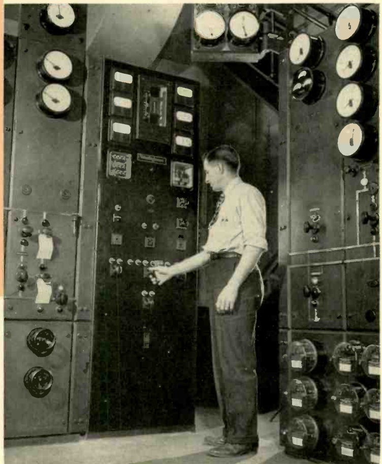
Fig. 2—The firing time of the ignitron tubes and hence the generator-field current is controlled by thyatrons. The method of regulating the thyatrons is shown here.
