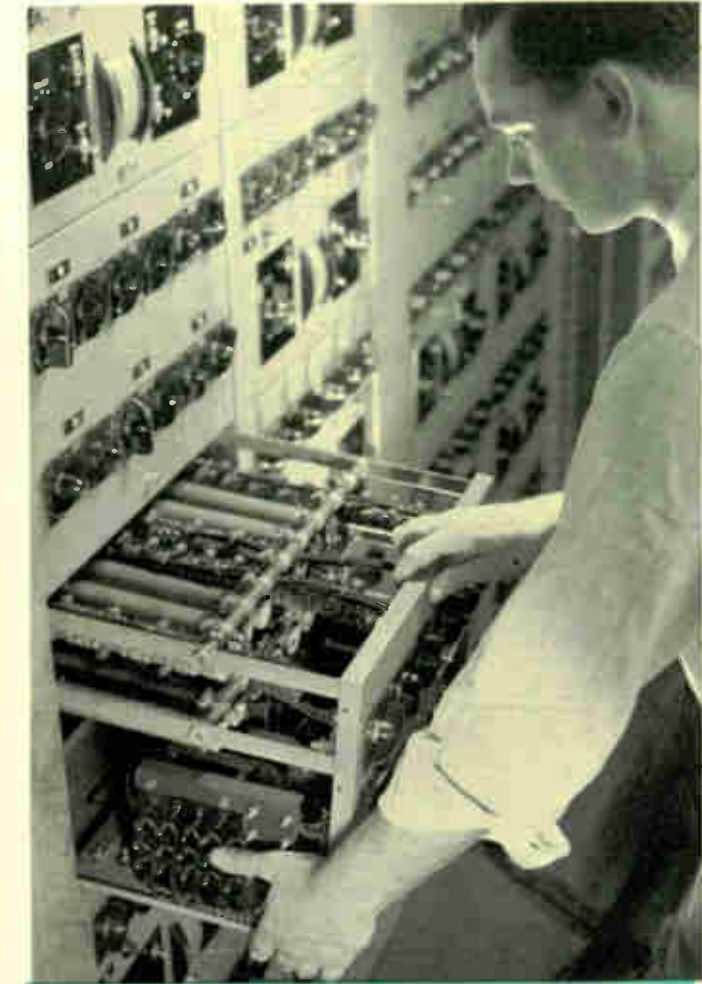
Each component of a power system has its electrical counterpart on the calculating board, such as this resistor-reactor unit.
