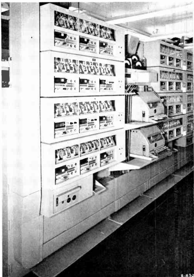
Figure 11. Sequence number indicator rack for line finder circuits
