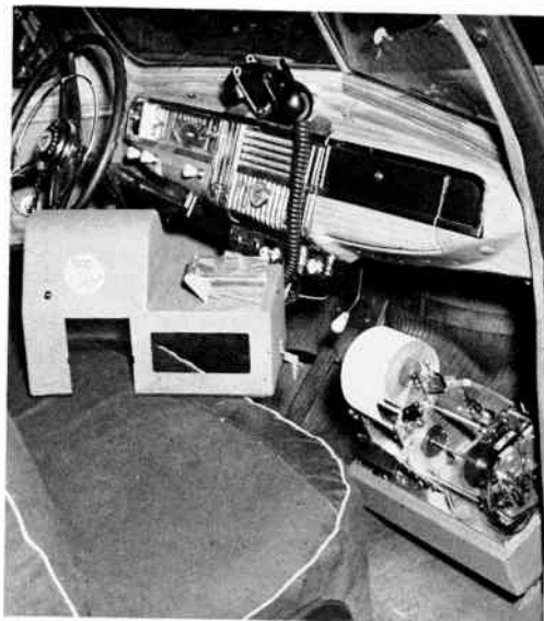
Figure 5. Facsimile recorder with cover removed
