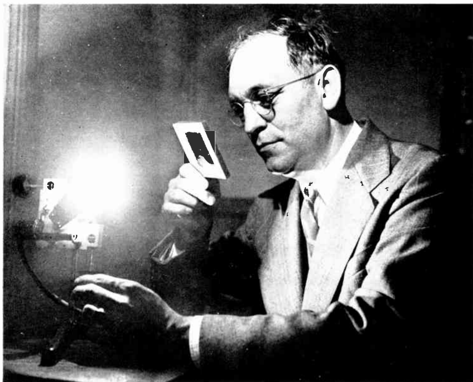
W. D. BUCKINGHAM of the Electronics Research Division with his invention, the Western Union Telcoarc. This is a further development of the zirconium arc lamp described in the April 1948 issue of TECHNICAL REVIEW ; both lamps are by-products of research on the use of modulated beamed light waves in communications. The new lamp burns in the open air and offers a highly concentrated source of brilliant light that can be useful in many fields outside of the telegraph industry. This Telcoarc development will be explained in detail in a future issue of the REVIEW .
