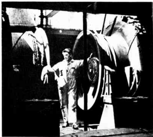
Figure 7. Cable handling machinery
